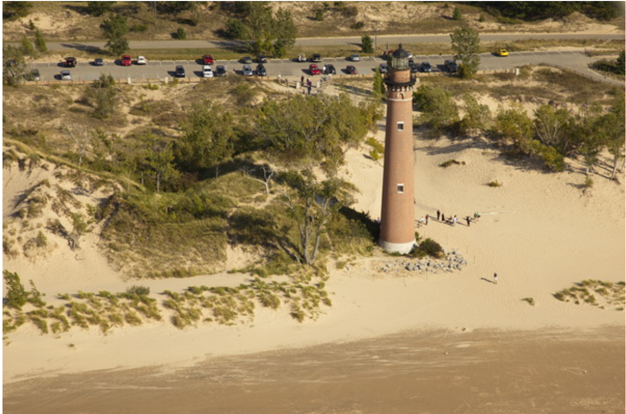
Aerial View of Little Sable Point Light, Golden Township, Oceana County, Michigan, September 2013. Photo Credit: Aerial Photography, John L. Wagner, East Lansing, Michigan.
