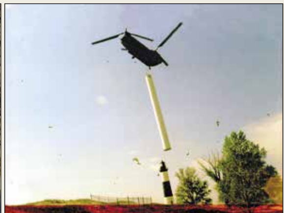
Helicopter picking up the D9 tower, 1996
