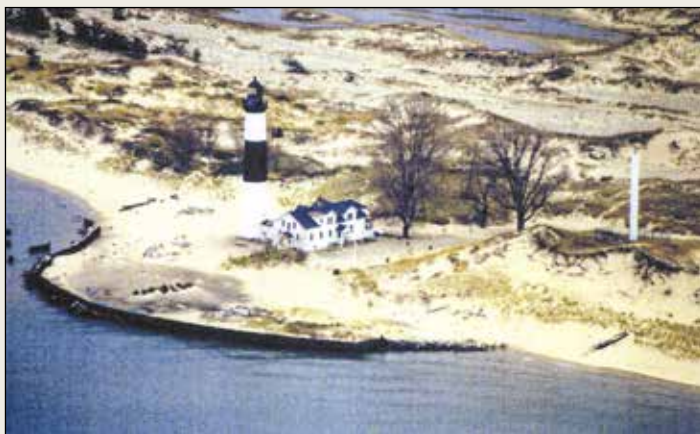
Late fall 1992 - with D9 tower still in place
