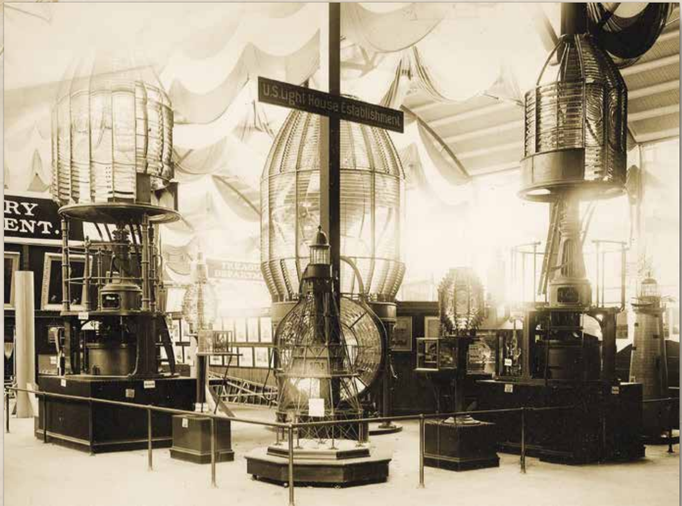
Scaled models of Fowey Rocks (center front) and Minot's Ledge (far right) lighthouses were displayed at the 1893 World's Columbian Exposition in Chicago along with a variety of lighting apparatus, including a hyperradial lens, first and second order Mahan system lenses, fourth order revolving lens, fifth order lens with occulting chimney, range lenses, 5-day and 8-day lens lanterns, light vessel lantern with lamps and reflectors, hand lanterns and electric buoy lanterns, some of which are shown in this photo. (National Archives)
