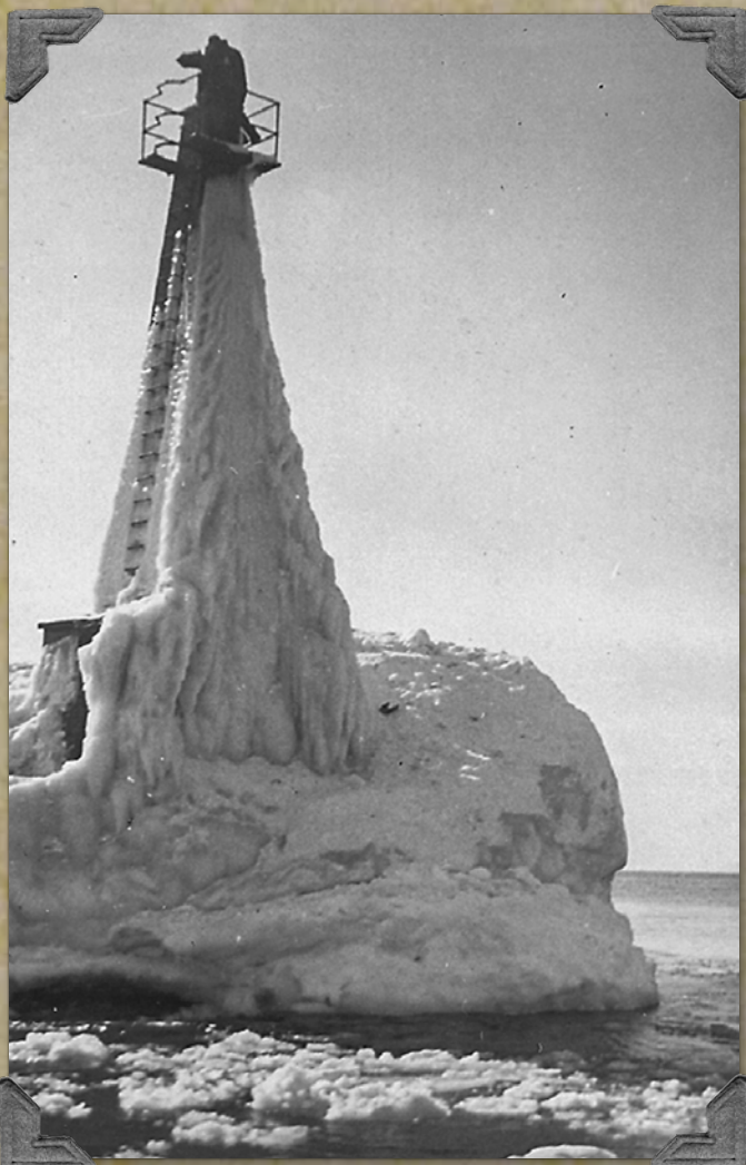
This 1935 photo of the 1920s Ludington South Breakwater Light shows how difficult it was to maintain in the winters. Fred had to chop ice off the steps to get to the top to relight it whenever high waves washed over it and doused the light. (Courtesy of Maribeth Schmock Runyan)
