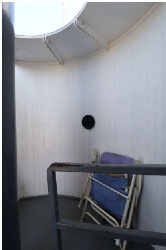
Figure 1D-316 Painted wood paneling and metal base in the Watch Room.
