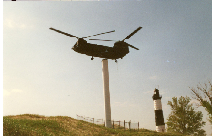
Figure 1B-100: 1996 photo of the pole tower being removed.
