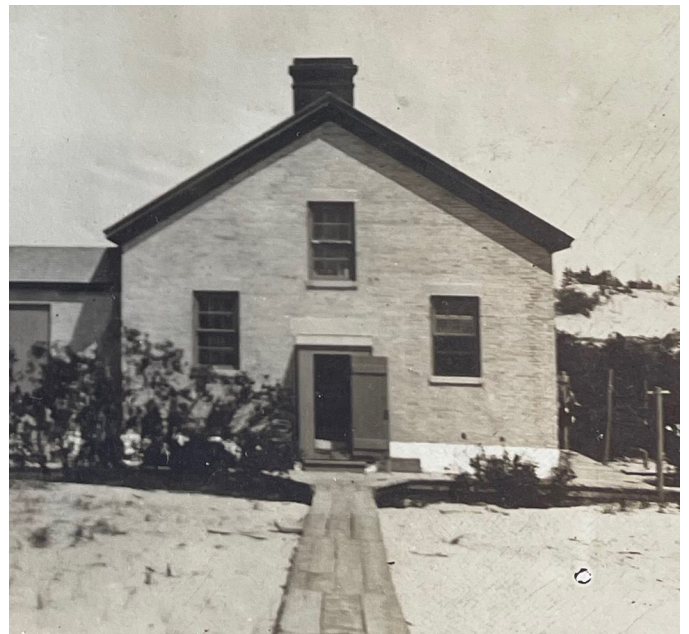
Figure 1B-06: 1900 photograph looking east at the keeper's dwelling.
