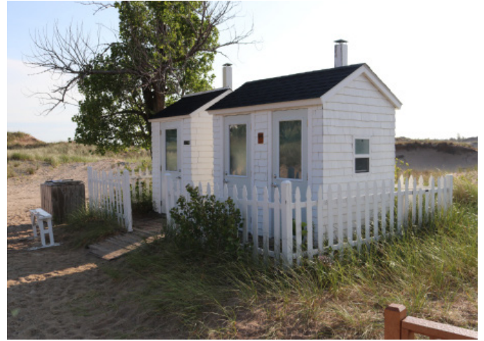
Figure 1D-12 West and north elevations of the public Vault Toilets.
