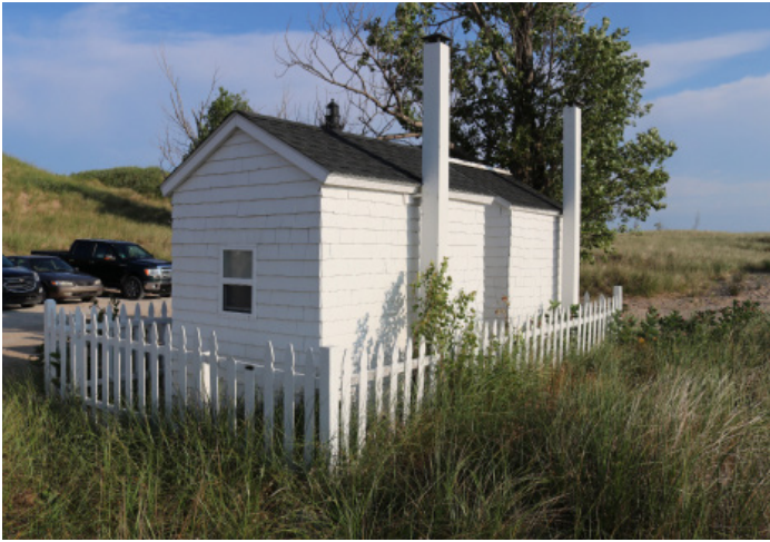
Figure 1D-11 South and east elevations of the public Vault Toilets.
