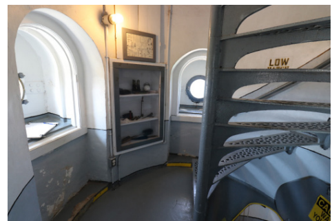
Figure 1D-313 Built in wood shelves at the fourth landing level.
