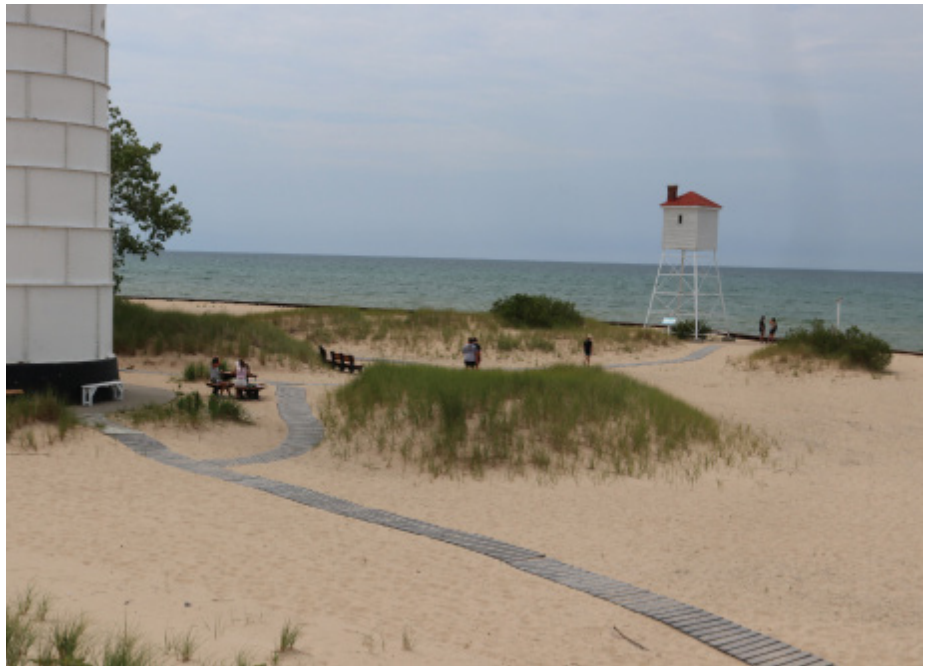
Figure 1D-21 Composite material plank sidewalks around the north side of the Light Tower.
