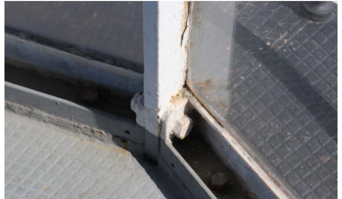
Figure 1D-326 Vertical mullion and base frame around Lantern glass.
