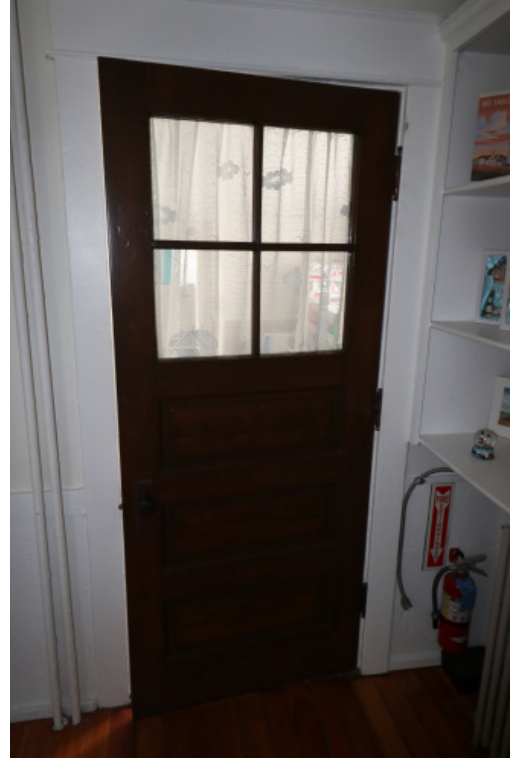
Figure 1D-111 Wood door at the entry to the Gift Shop from the North Porch.
