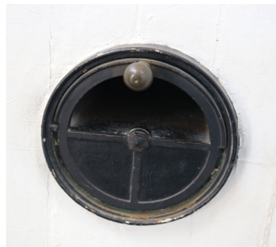
Figure 1D-318 Lantern ventilator, interior view.
