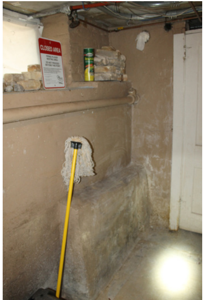
Figure 1D-45 Underpinning present in north brick masonry foundation wall.
