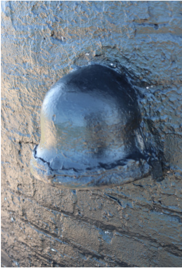
Figure 1D-319 Lantern ventilator, interior view.
