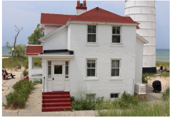
Figure 1D-37 East elevation of the Keepers' Dwelling.
