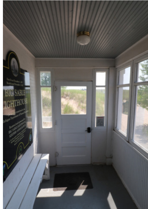
Figure 1D-108 Wood door at the southeast porch.
