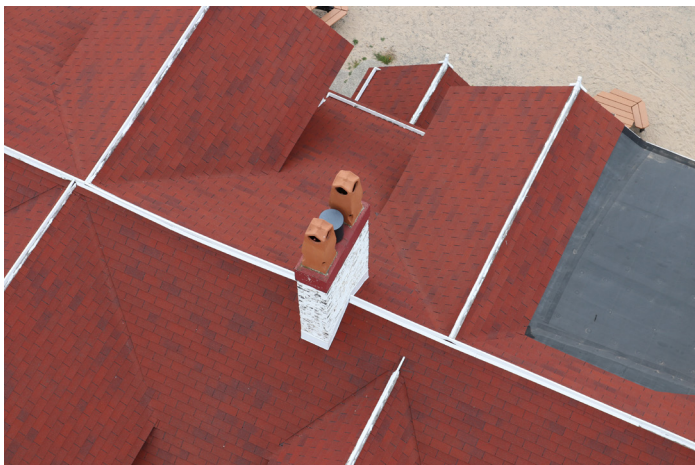
Figure 1D-90A View of chimney from the Light tower.
