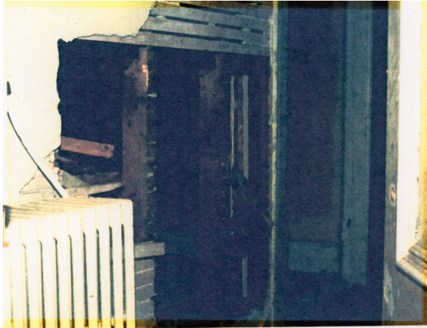
Figure 1B-77: Undated photo showing a section of wall that was removed.
