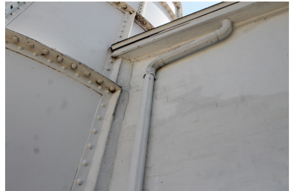
Figure 1D-225 Cracking present at north end of west wall at intersection of tower.
