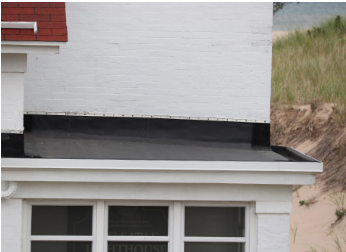
Figure 1D-85 EPDM roof on the Southeast Porch.
