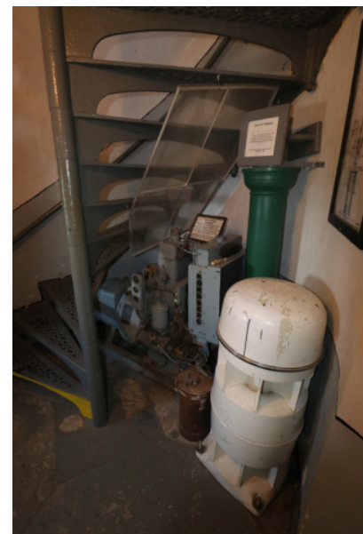
Figure 1D-309 Navigation aids stored below the Light Tower stair.
