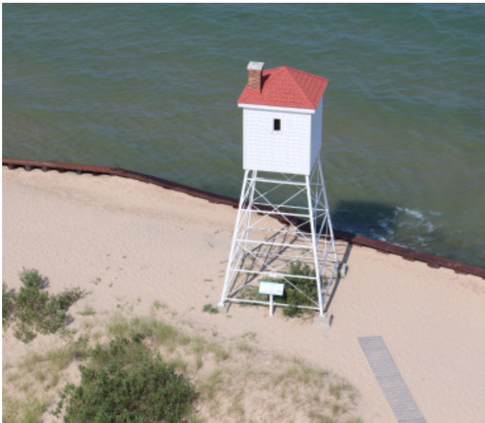
Figure 1D-29 Fog Signal Tower as viewed from the Light Tower.
