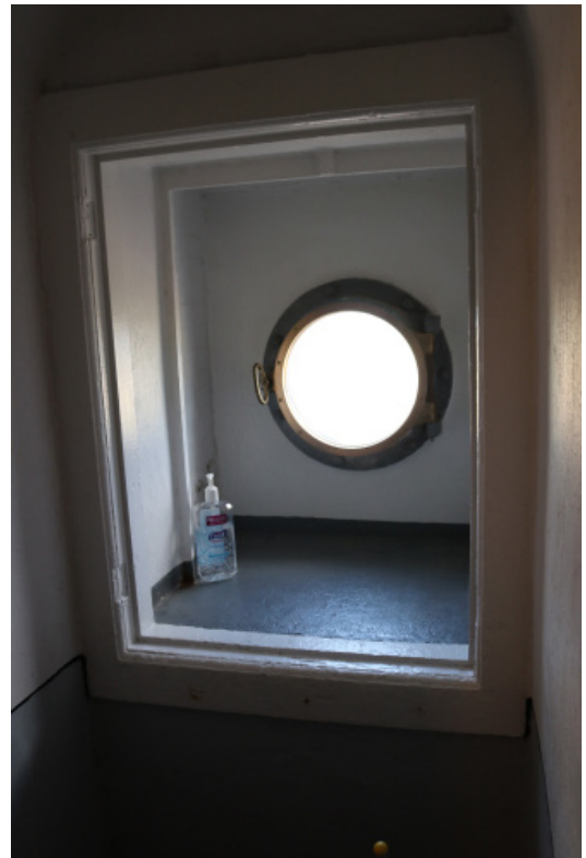
Figure 1D-282 Interior view of Porthole window and non-extant original rectangular tower window.
