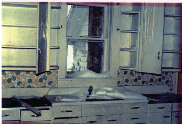
Figure 1B-78: Undated photo showing snow accumulating in the kitchen at a broken window.
