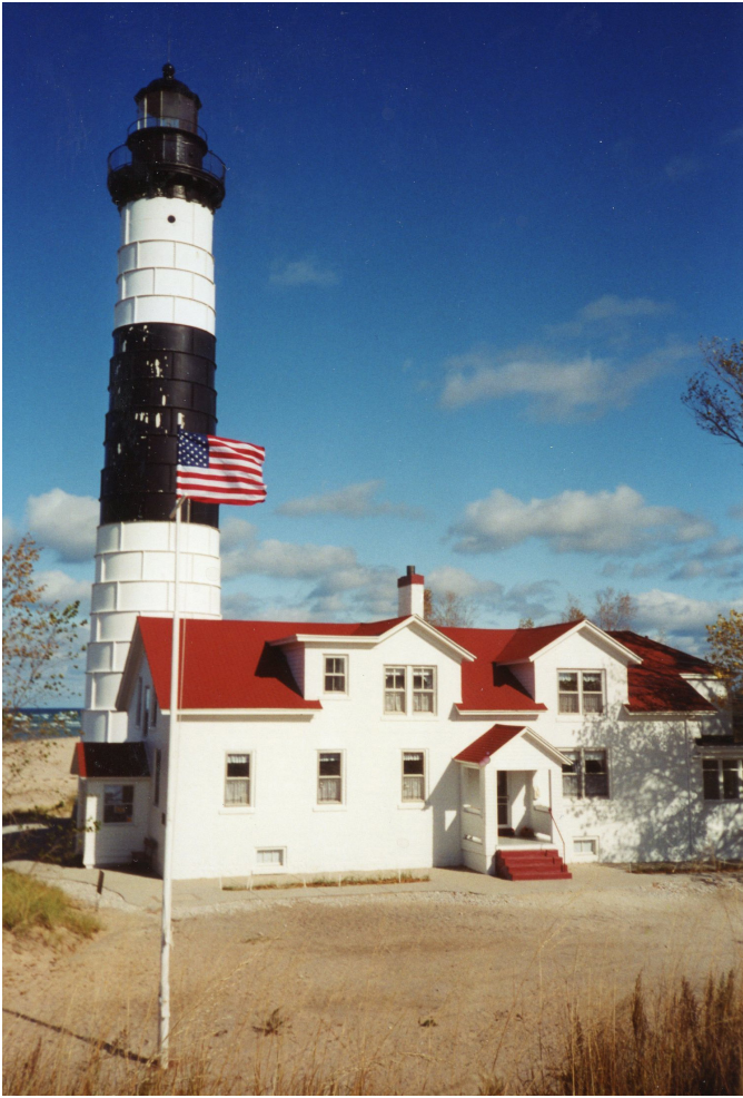
Figure 1C-30: Circa late 1990s photo looking northeast toward the Keepers' Dwelling showing the replacement concrete walkways.
