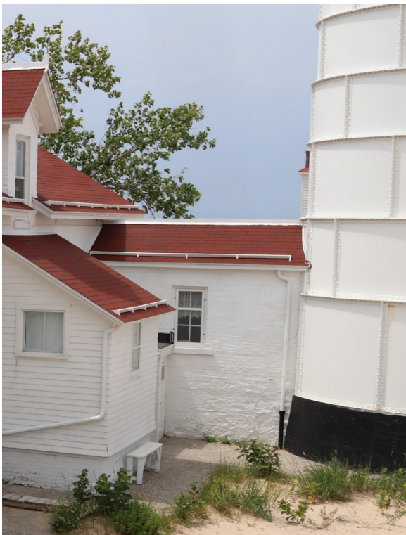
Figure 1D-231 East wall of the Passageway with single window.
