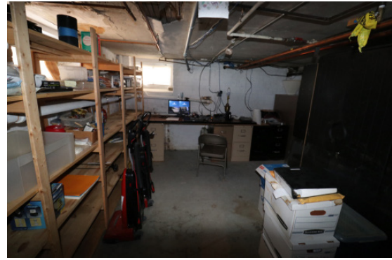
Figure 1D-184 Security Room, with security equipment and monitors, in the east part of the Basement.
