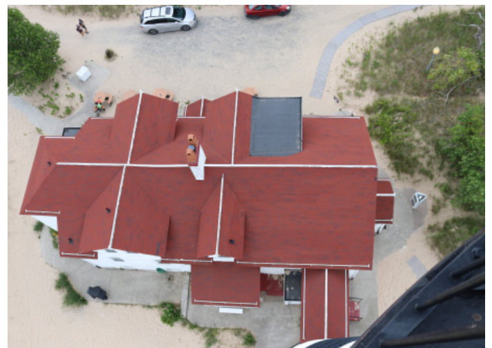
Figure 1D-83 Asphalt shingle roof of the Keepers' Dwelling and Passageway as seen from the Light Tower.
