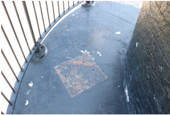
Figure 1D-295 Cast iron floor of the Watch Deck.
