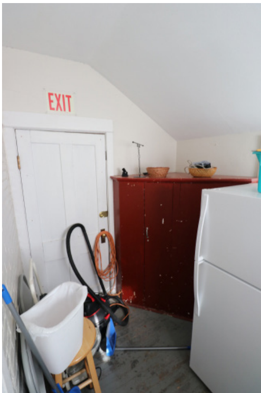
Figure 1D-112 Wood door at the entry to the North Porch.
