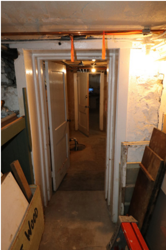
Figure 1D-193 Painted wood door in the Basement through the wall connecting the east and west parts.
