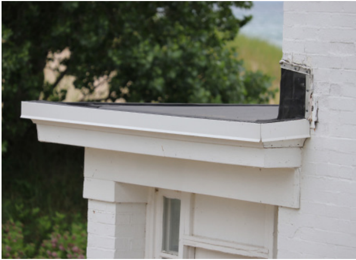
Figure 1D-84 EPDM roof on the Southeast Porch.
