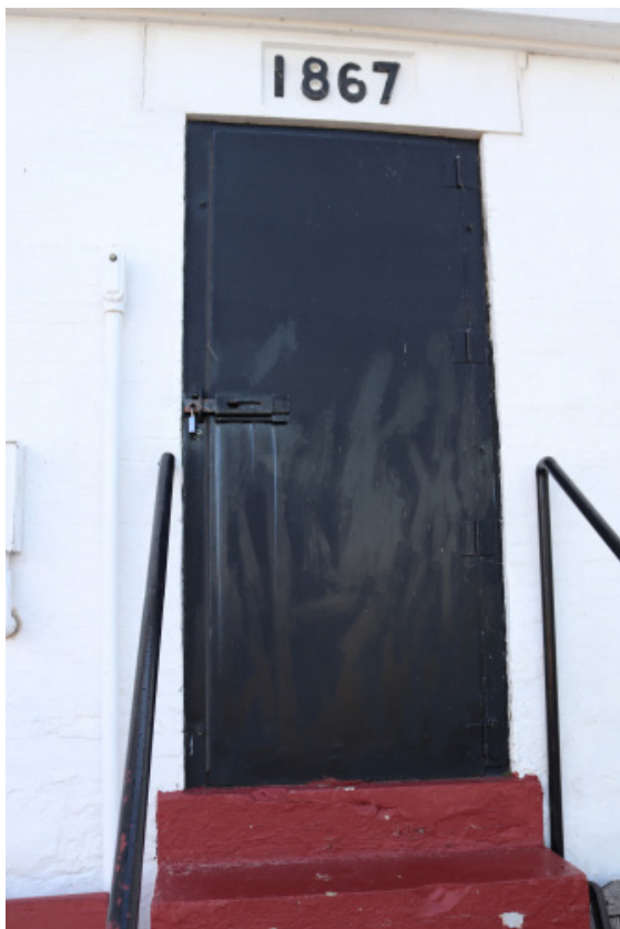
Figure 1D-234 Steel plate door on the west wall of the Passageway.
