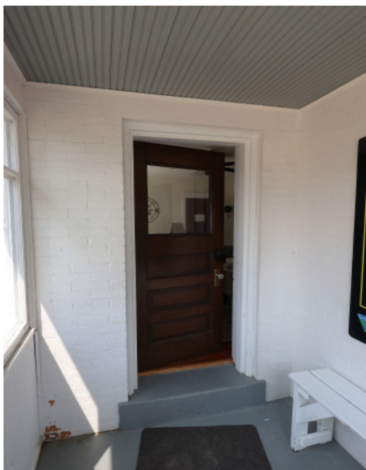
Figure 1D-123 Southeast porch and entry door into the apartment. Note step up at door.
