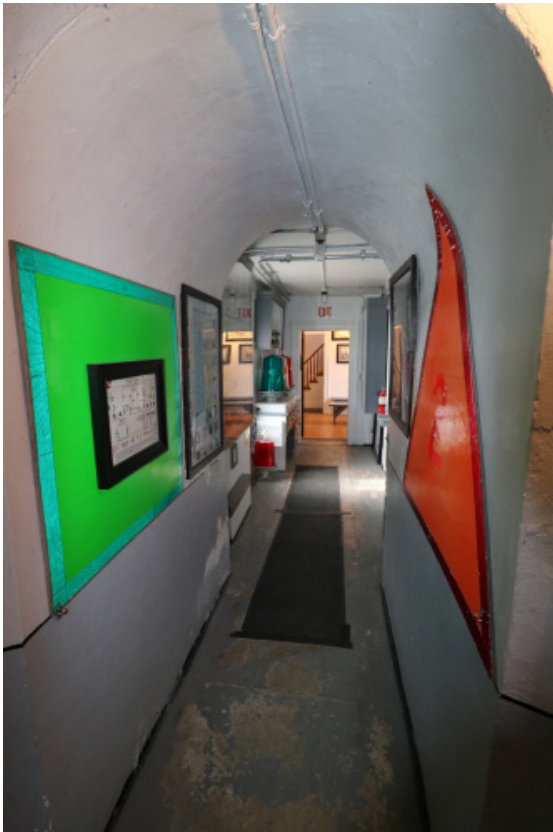
Figure 1D-237 Interior view of Passageway from within the Light Tower walls.
