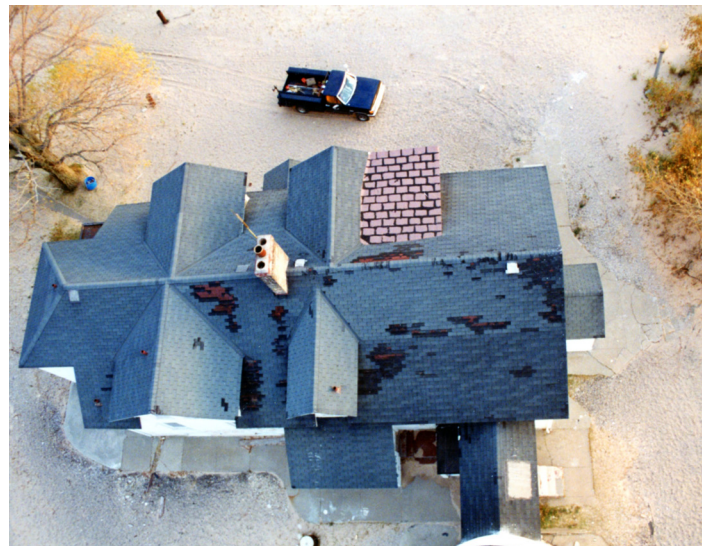
Figure 1C-29: Circa 1980s photo looking down at the Keepers' Dwelling from the tower.
