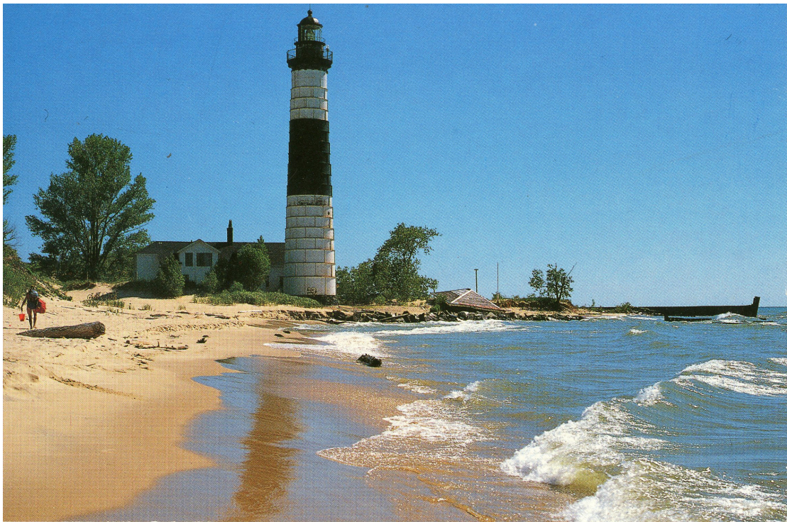
Figure 1B-87: Summer 1982 photo looking southwest toward the station buildings. The fog signal control building has collapsed. Concrete from the structure was used as rip rap shore protection.
