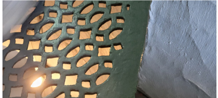
Figure 1D-261 Casting defect along edge of lattice work in tread.
