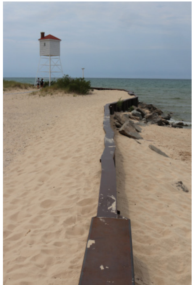
Figure 1D-33 Steel sheet pile breakwater and stone rip-rap.
