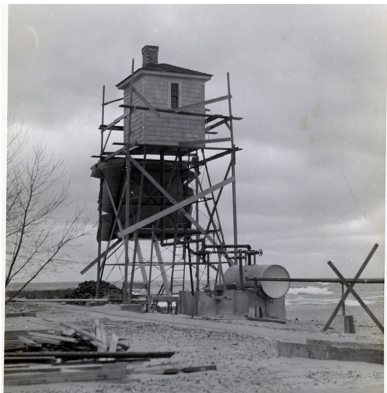
Figure 1B-49: Photo of the fog signal tower under construction.
