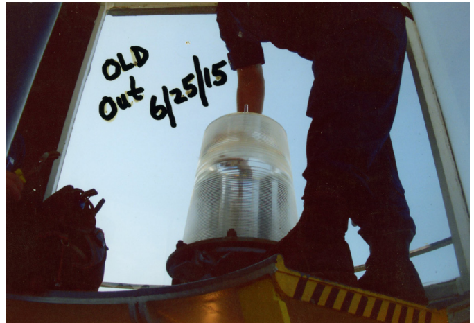
Figure 1A-09: 2015 photo of the plastic lens being removed.
