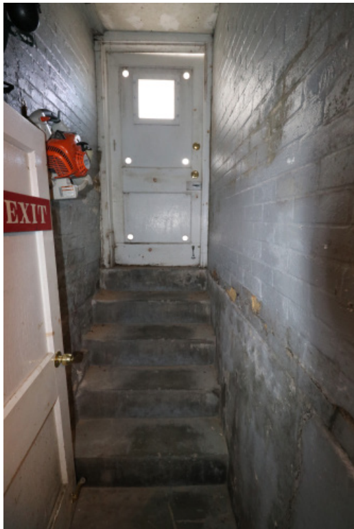
Figure 1D-115A Wood door at the Basement stairwell on the north elevation.
