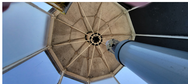
Figure 1D-254 Roof structure exposed in lantern room.
