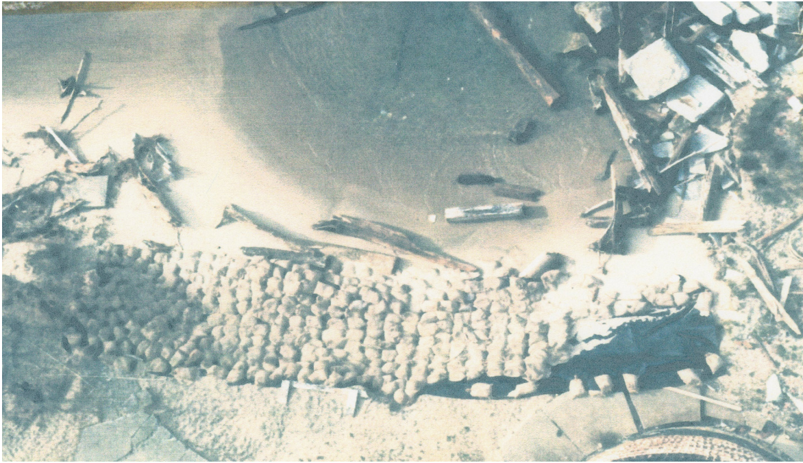
Figure 1C-35: November 1986 photo showing sandbags being installed north of the tower.
