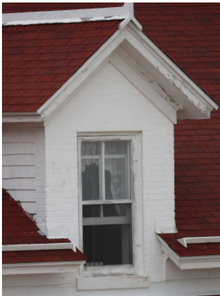
Figure 1D-106 Second floor double hung window.
