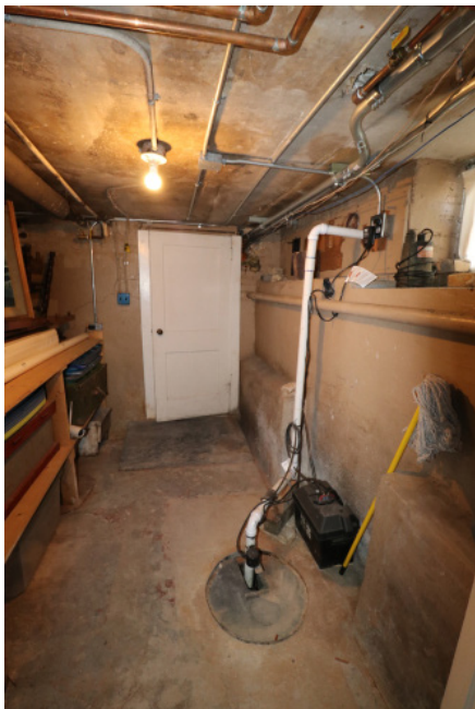
Figure 1D-183 Storage Room in the east part of the Basement.
