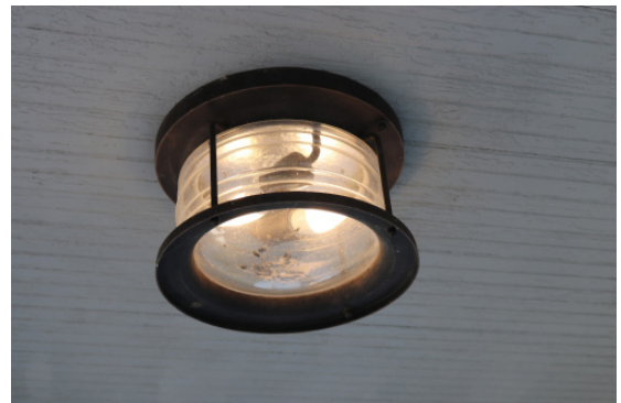
Figure 1D-218 Interior light fixture example.
