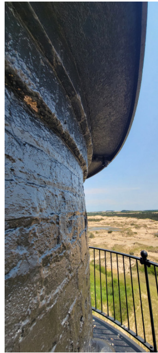
Figure 1D-264 Coated brick on exterior of tower above lantern floor balcony.
