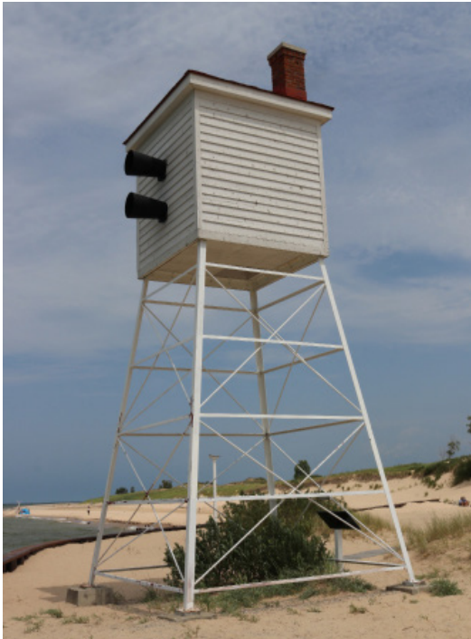
Figure 1D-31 South and west elevation of the Fog Signal Tower.
