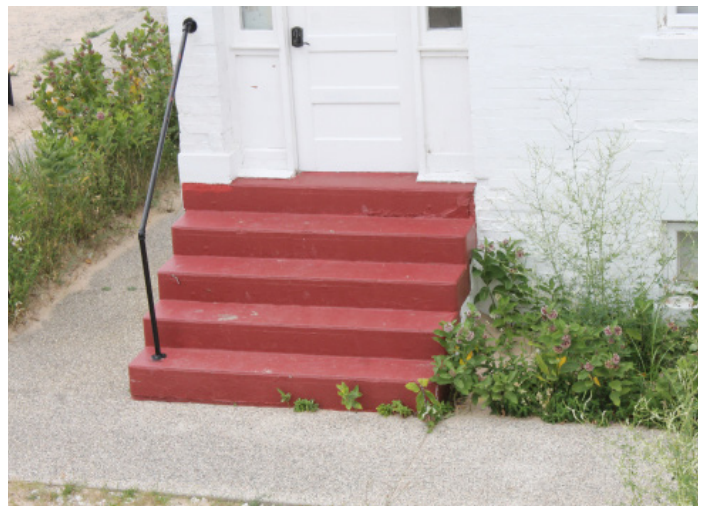
Figure 1D-81 East stairs up to first floor level of Keepers' Dwelling.
