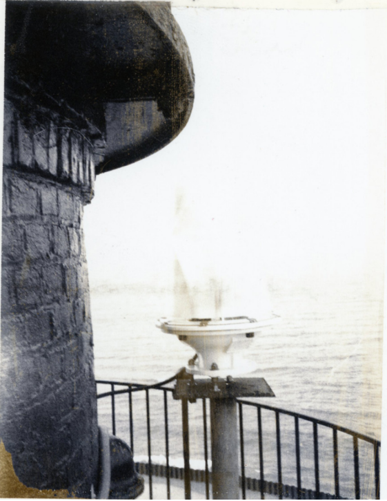
Figure 1B-75: Photo of the stand-by light installed on the lantern gallery in 1971
