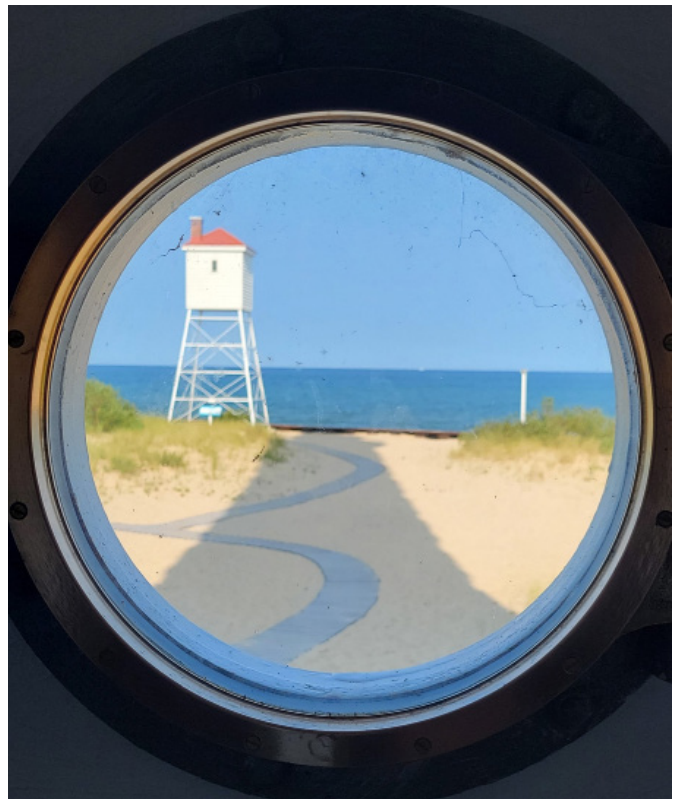
Figure 1D-03 Fog signal tower replica south of the shadow of the light tower, as viewed through the light tower portal at grade.
