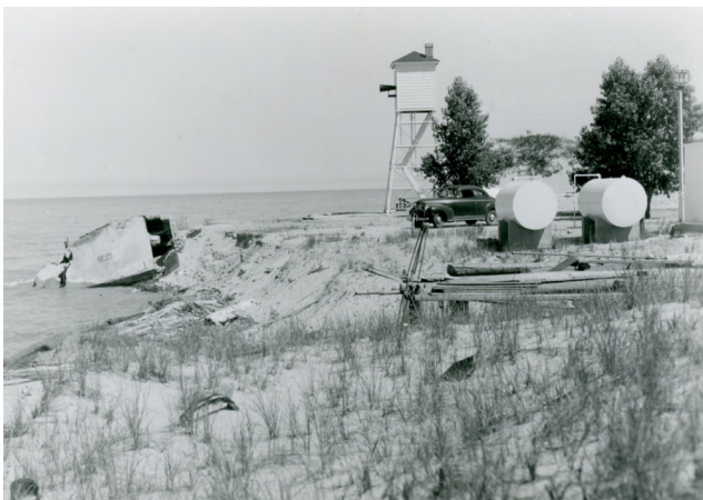
Figure 1B-53: 1943 photo of the collapsed remaining portion of the fog signal building in the water.
