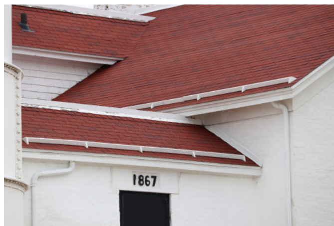
Figure 1D-229 Asphalt shingle roof on the Passageway.
