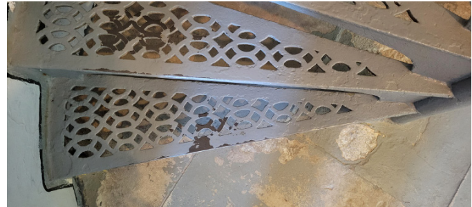
Figure 1D-256 Top view of latticed stair tread.
