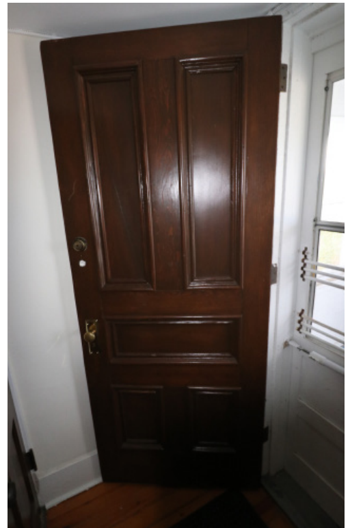
Figure 1D-113 Wood door at the Gift Shop entry from the West Porch.
