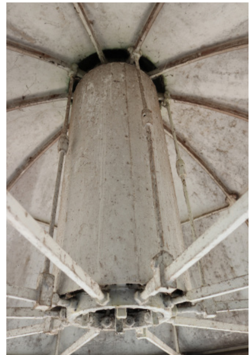
Figure 1D-328 Lantern chimney.
