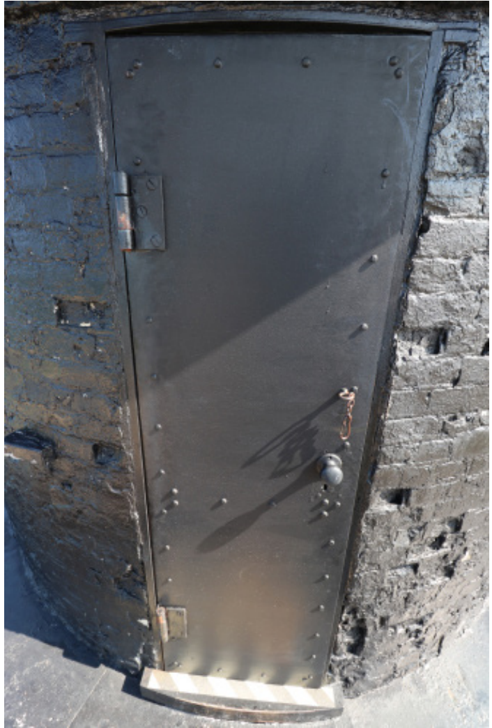
Figure 1D-289 Exterior steel plate door providing access from the Watch Room to the exterior Watch Deck.
