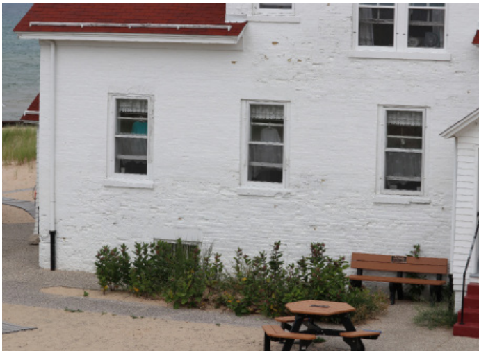
Figure 1D-93 Detail of the painted brick masonry on the south elevation.
