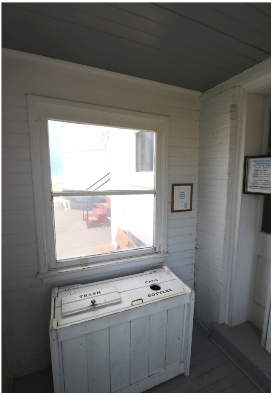
Figure 1D-145 Enclosed Porch on the west elevation leading to the Gift Shop entry.
