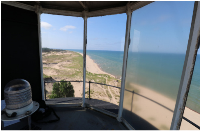
Figure 1D-323 Lantern glass panels looking south.
