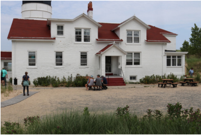
Figure 1D-36 South elevation of the Keepers' Dwelling.
