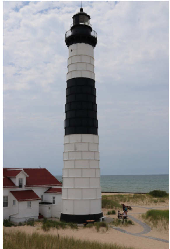
Figure 1D-244 North/northeast elevation of the Light Tower.
