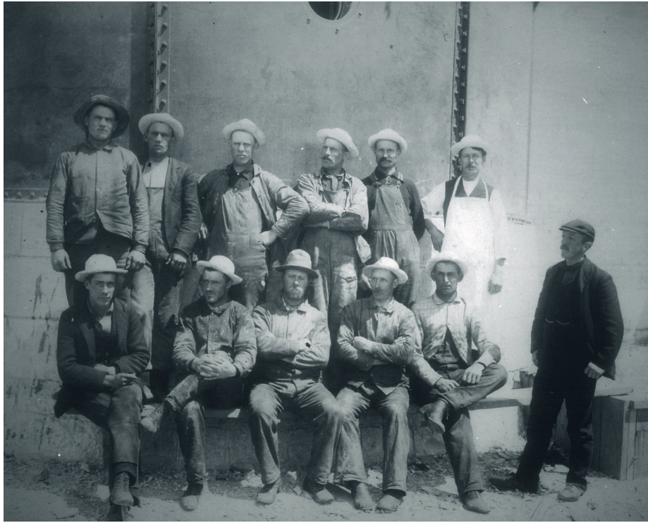
Figure 1B-14: 1900 photograph of the construction crew that encased the tower in metal plates.
