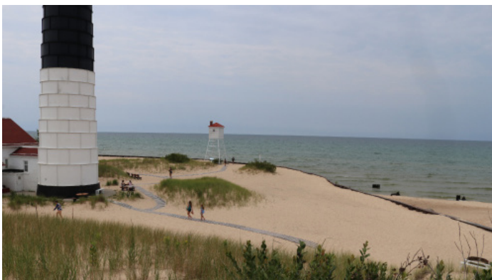
Figure 1D-32 Steel sheet pile breakwater.
