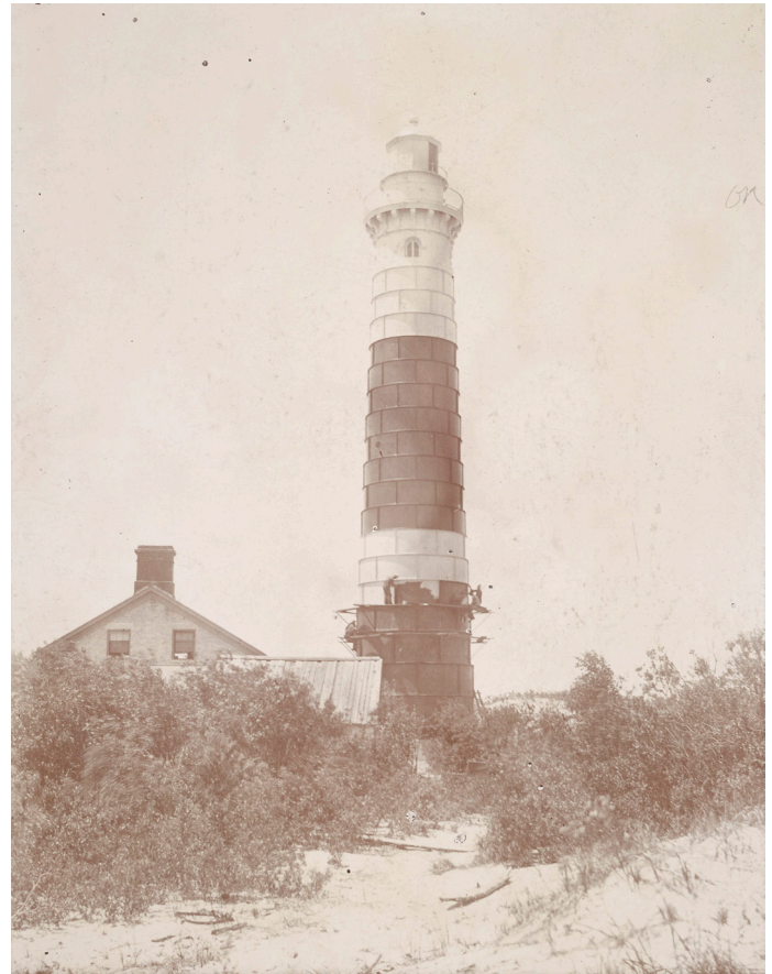
Figure 1B-16: 1900 photograph looking west at the new metal plating at the tower being painted. The roof of the one-story portion of the keeper's dwelling and the barn that may have housed the original construction crew can also be seen in this photo.
