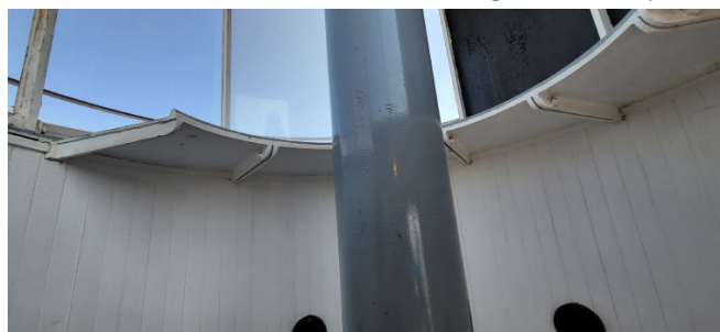
Figure 1D-253 Upper walkway of lantern room floor.
