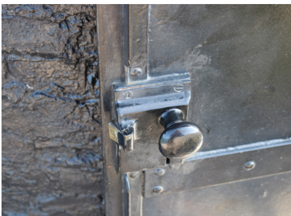
Figure 1D-291 Steel plate door hardware.
