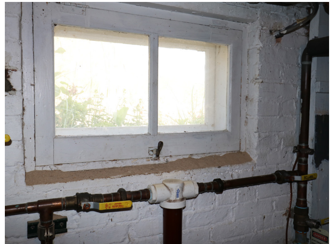
Figure 1D-97 Interior view of typical in-swinging, top hinged Basement window.
