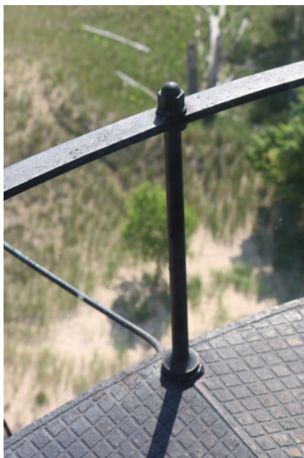
Figure 1D-303 Top rail and post at the Lantern Deck railing.
