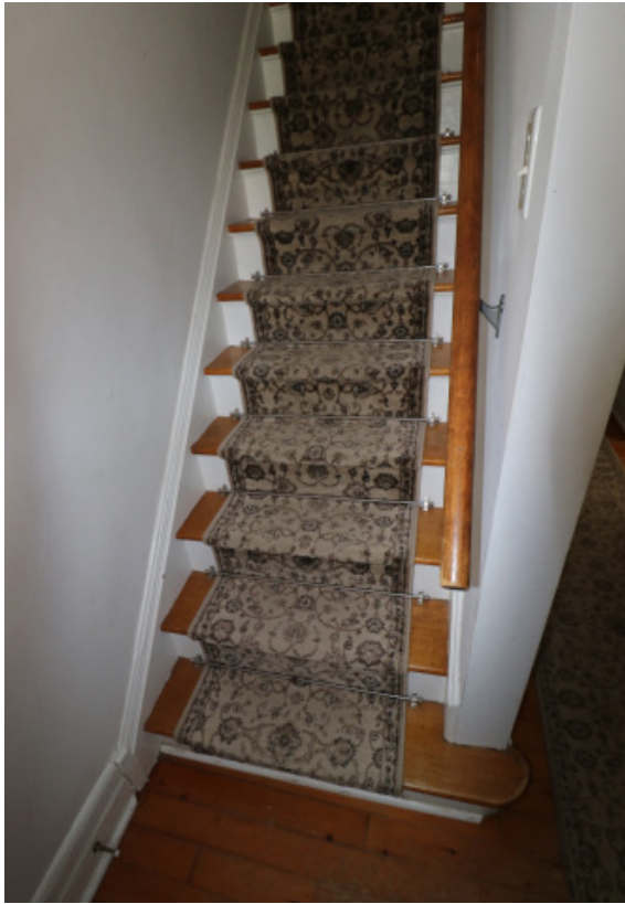
Figure 1D-128 Lower section of the stairway leading to the second floor apartment.
