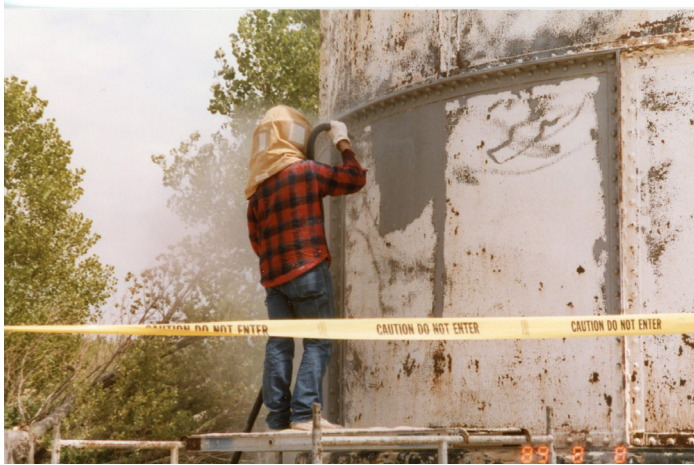
Figure 1B-94: 1989 photo taken during the 1989 tower repairs showing a section of the metal cladding being welded.
