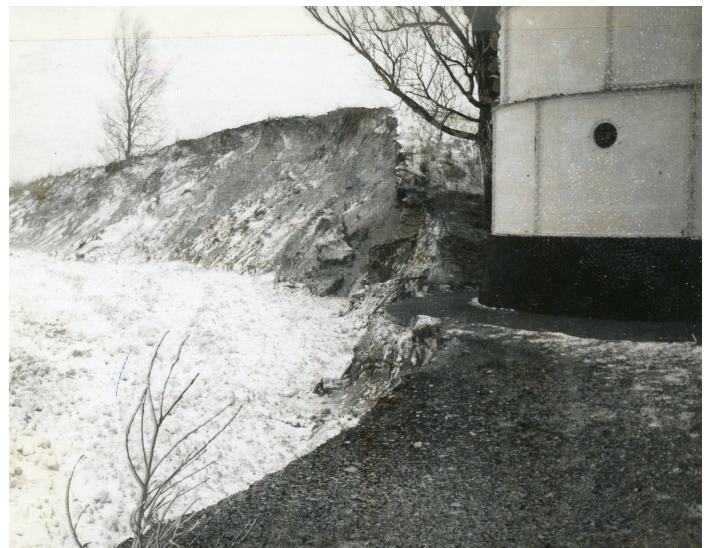
Figure 1B-85: 1978 photo showing shoreline erosion up to concrete sidewalk around the tower base. The handwritten caption on the back of the photos says, "Photo taken from west side of Lt. Tower. Erosion cutting close. Concrete walls is 7' above beach, and 8.5' above water line. Slush covers entire area."
