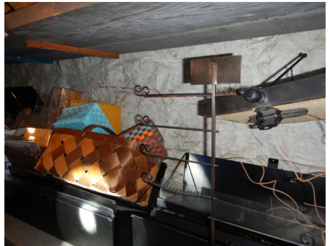
Figure 1D-41 Step cracking in center stone masonry bearing wall behind storage shelves.
