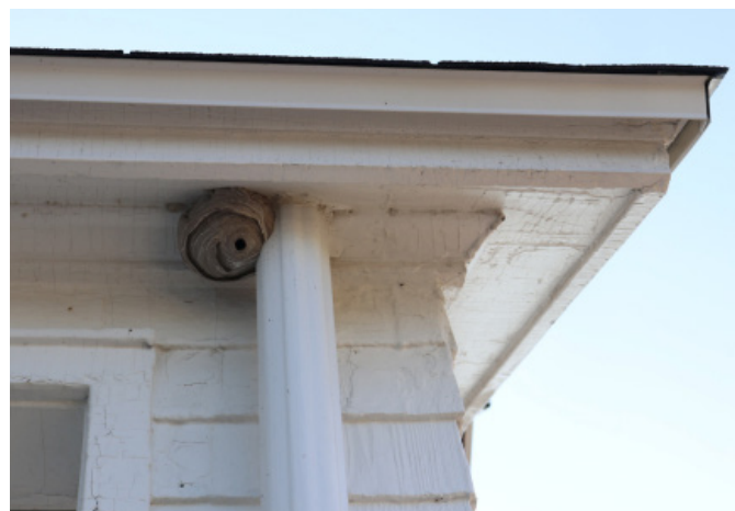
Figure 1D-92 Non-active metal gutter terminating in the soffit.
