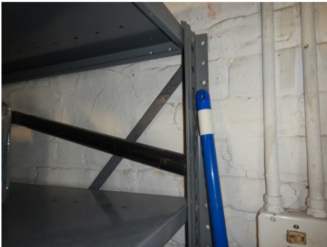
Figure 1D-44 Minor step cracking in brick masonry center bearing wall.
