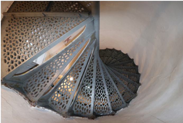
Figure 1D-310 Inner tower plaster walls and circular stair.
