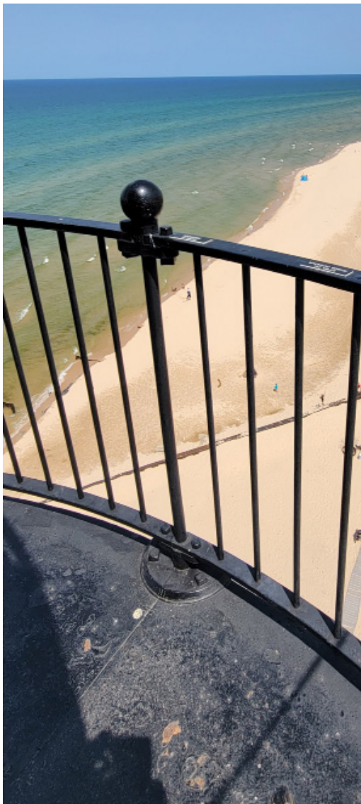
Figure 1D-274 Exterior metal railing at the Watch Deck level.
