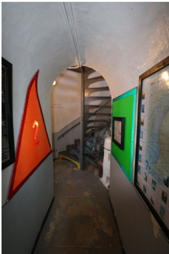
Figure 1D-238 Interior view of Passageway looking towards the circular stair of the Light Tower.
