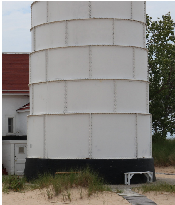
Figure 1D-279 Painted "black" stone masonry base of the Light Tower.
