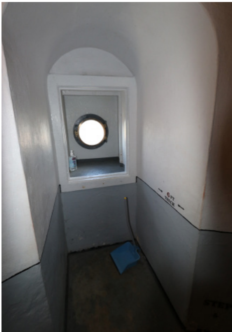
Figure 1D-308 Light Tower window at main floor level.
