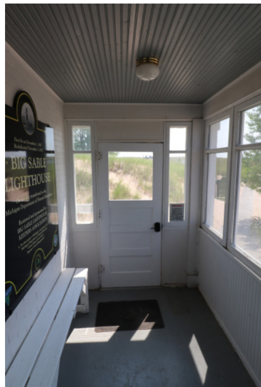
Figure 1D-122 Porch on the southeast corner leading to the first floor apartment entry.
