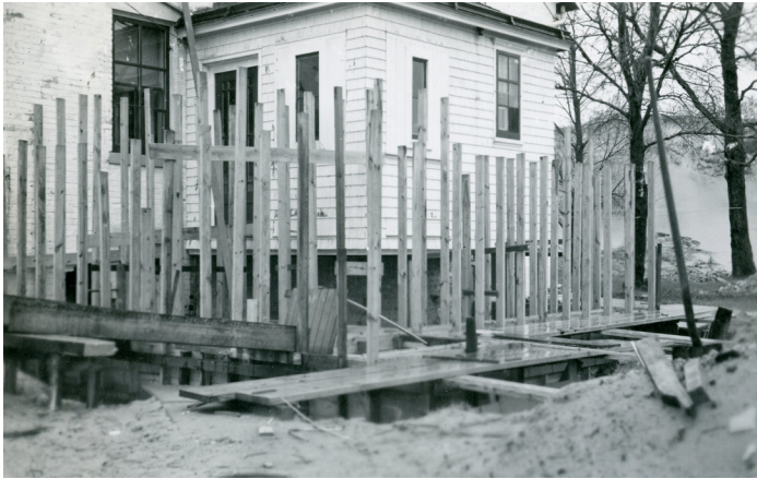
Figure 1B-70: Construction photo of the keeper's dwelling addition.
