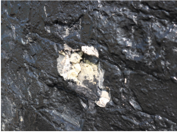
Figure 1D-288 Deteriorated paint surface and damaged brick on the exterior brick masonry wall at the Watch Deck.
