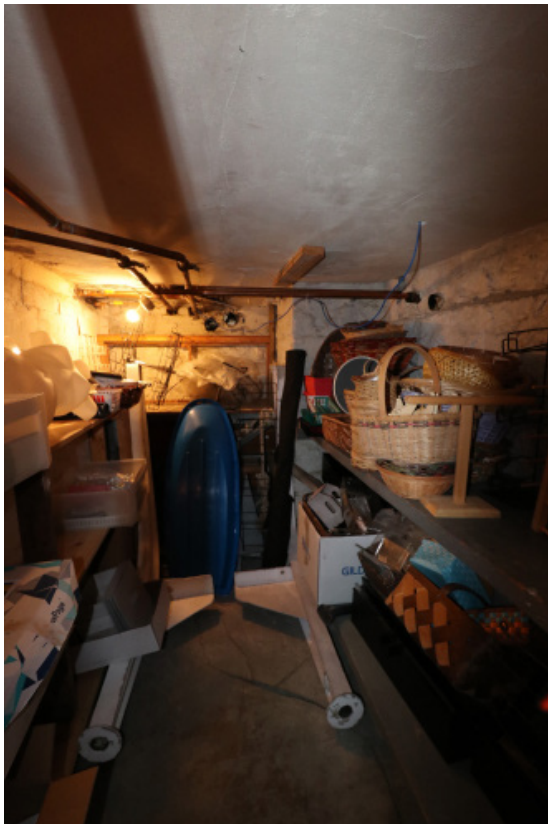
Figure 1D-190 Storage Room constructed of concrete masonry unit walls.
