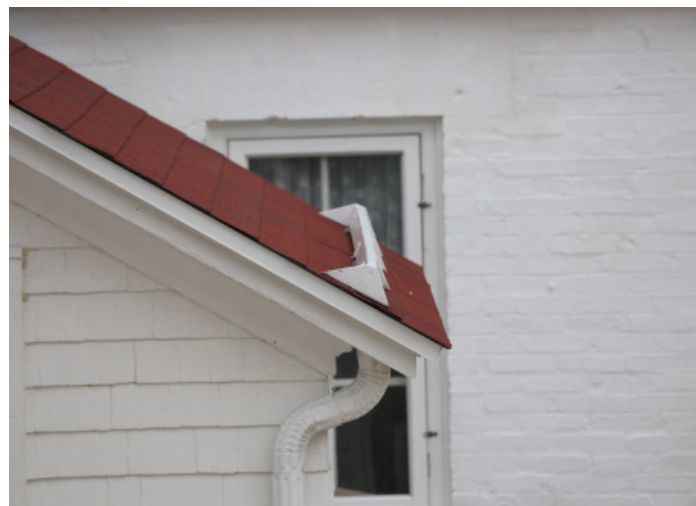
Figure 1D-91 Non-active metal gutter terminating in the soffit.
