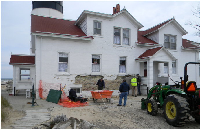
Figure 1B-106: Photo taken during the 2013 masonry workshop.
