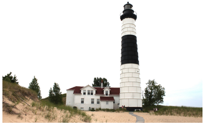
Figure 1D-01 Overall Keepers' Dwelling north elevation.
