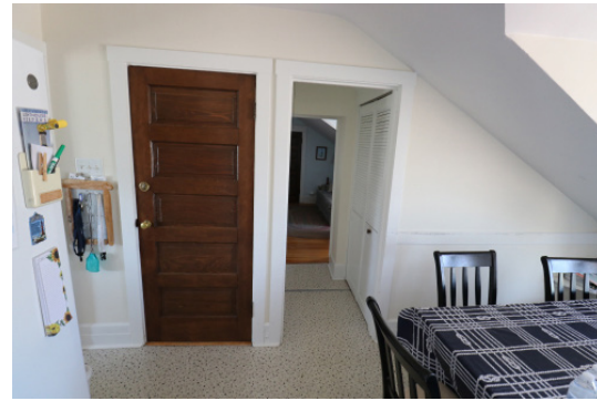
Figure 1D-172 Interior wood panel door and painted wood louver Pantry door in the second floor Hallway.
