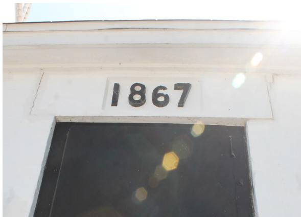
Figure 1D-223 No visible displacement of connector link roof structure, misalignment and cracking present on either side of stone masonry header.
