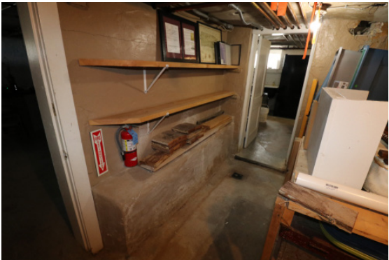
Figure 1D-182 Storage Room in the east part of the Basement.
