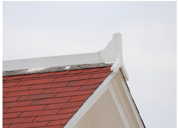
Figure 1D-88 Decorative wood ridge boards.
