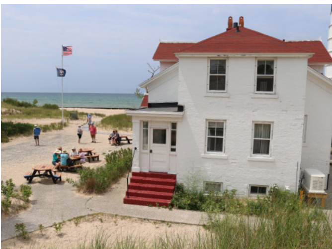
Figure 1D-19 Concrete sidewalks around the Keepers' Dwelling.
