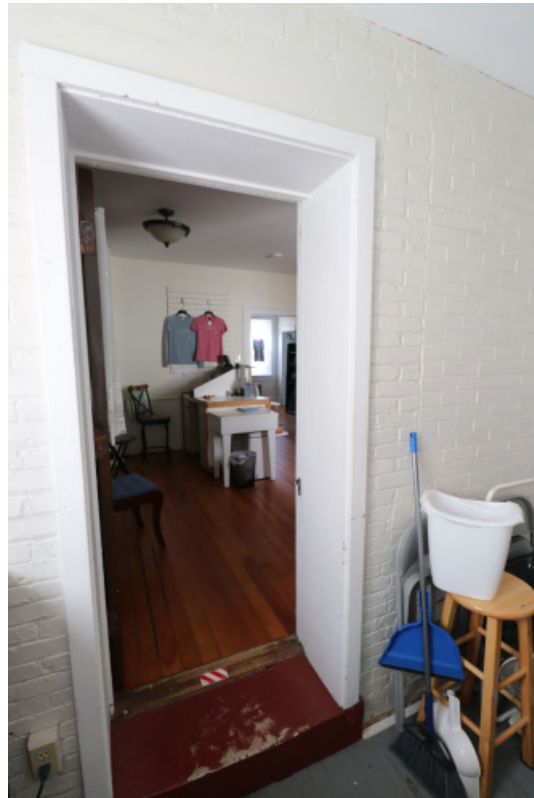
Figure 1D-147 Door opening in the masonry wall between the North Porch and the Gift Shop.
