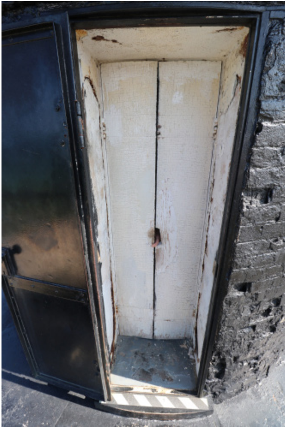
Figure 1D-293 Exterior face of the pair of inner wood doors.
