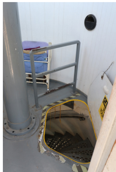
Figure 1D-315 Metal guardrail and navigation light pedestal protecting the floor hatch opening.
