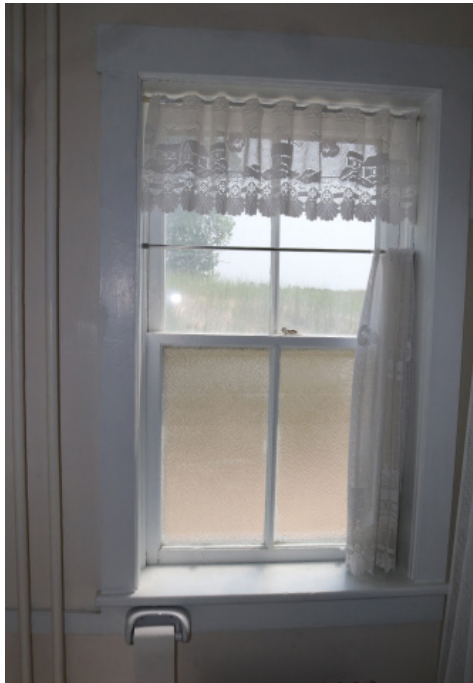
Figure 1D-100 Interior view of first floor Bathroom double hung window on the east elevation.
