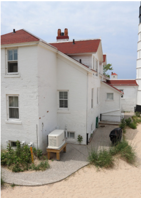
Figure 1D-20 Concrete sidewalks around the Keepers' Dwelling.
