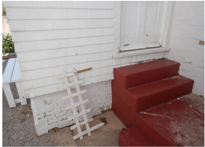
Figure 1D-80 North stairs up to first floor level of Keepers' Dwelling.
