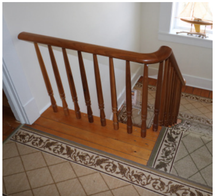
Figure 1D-144 Stairway railing detail on the second floor.
