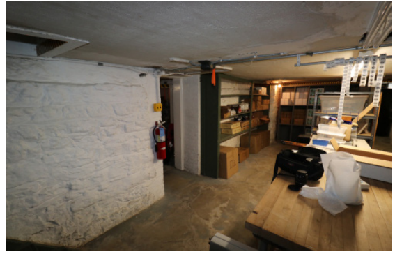
Figure 1D-187 General Storage Room in the west part of the Basement, north side.
