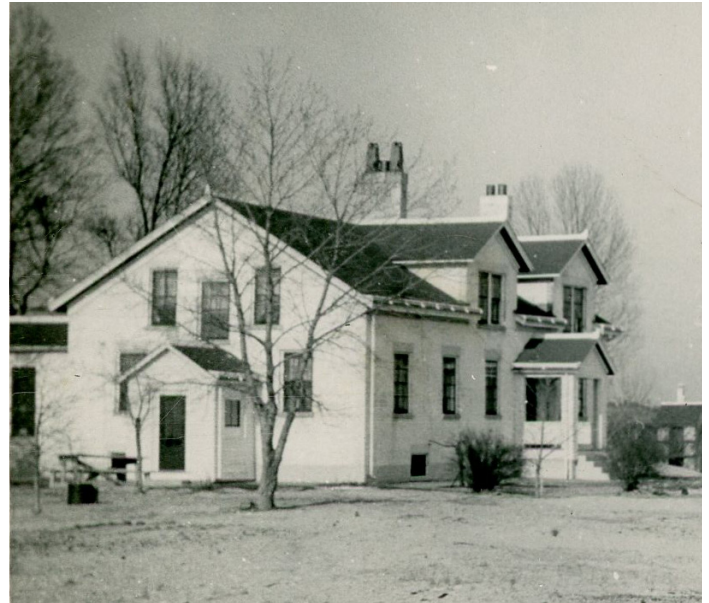
Figure 1C-03: Circa 1940s photo of the Keepers' Dwelling.
