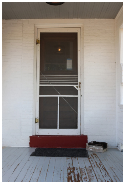
Figure 1D-109A Wood screen door at the south entry.
