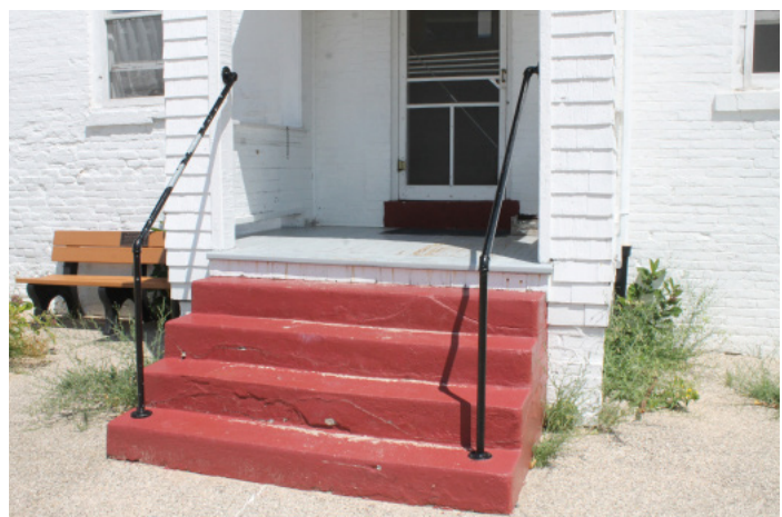
Figure 1D-82 South stairs up to first floor level of Keepers' Dwelling.
