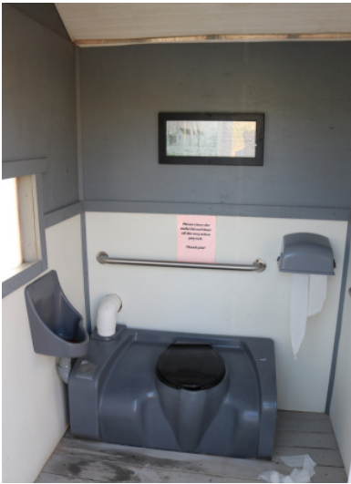
Figure 1D-13 Interior of Vault Toilet.
