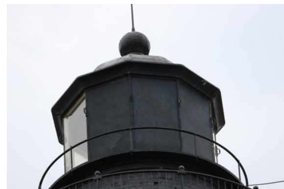
Figure 1D-301 Ten-sided Lantern.
