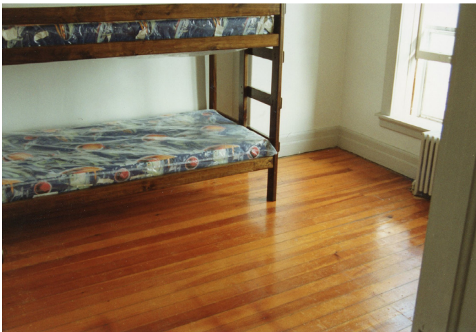
Figure 1B-99: 1991 photo of restored wood flooring.
