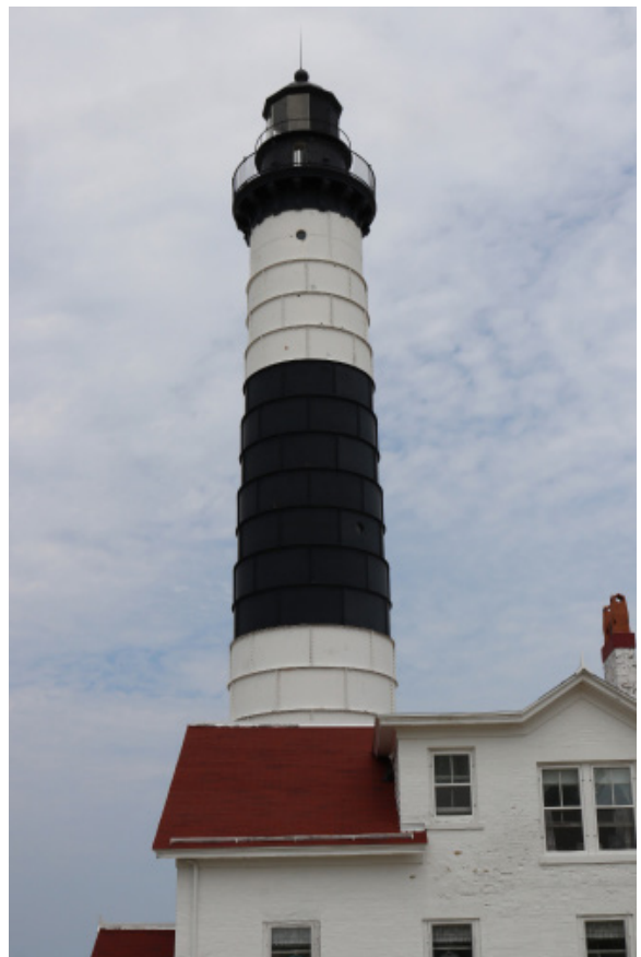
Figure 1D-246 South elevation of the Light Tower.
