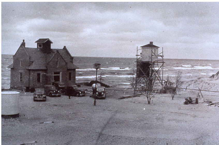
Figure 1B-50: Photo of the fog signal tower under construction northeast of the fog signal building.
