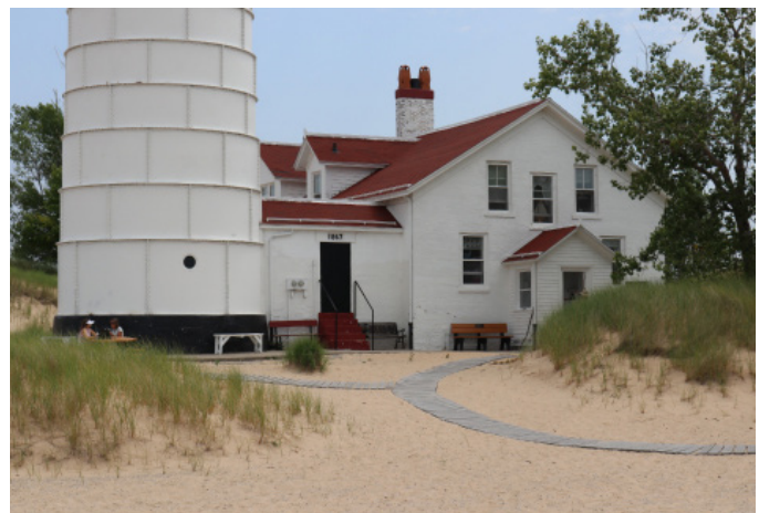
Figure 1D-35 West elevation of the Keepers' Dwelling.
