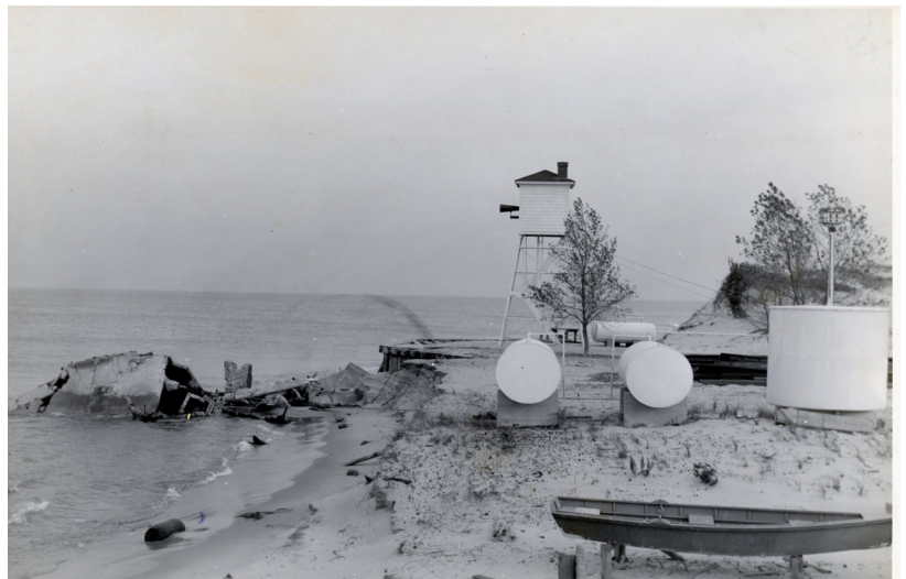
Figure 1B-54: 1943 photo of the collapsed remaining portion of the fog signal building in the water.
