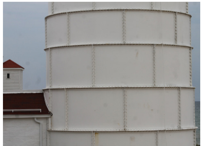
Figure 1D-265 General condition of east portion of tower metal cladding, note staggered alignment of vertical edges of plates creating an enlarged “running bond pattern” of the cladding.
