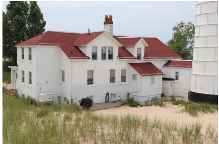
Figure 1D-34 North elevation of the Keepers' Dwelling.
