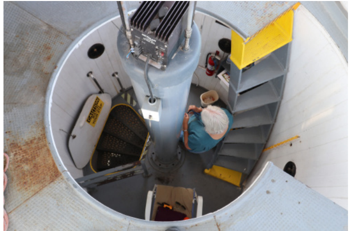
Figure 1D-321 View from Lantern looking down into the Watch Room. Note lack of guardrails around the floor opening.
