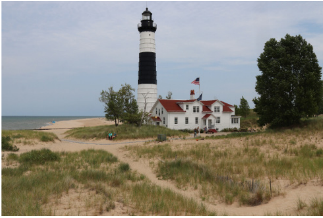
Figure 1D-04 View of the site looking north towards the light station.
