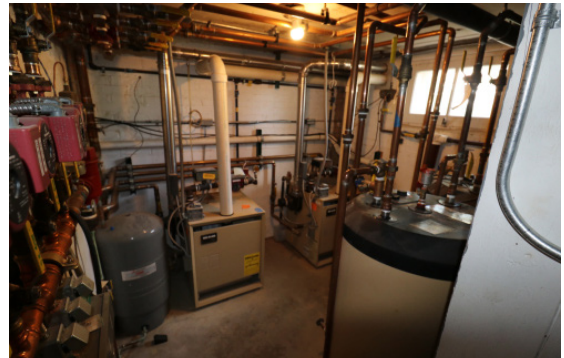
Figure 1D-179 Mechanical Room in the east part of the Basement.
