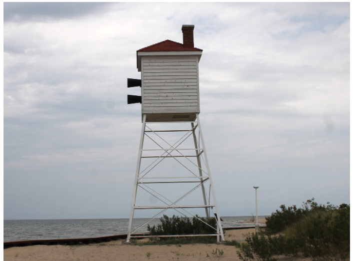
Figure 1D-334 Fog signal south elevation.
