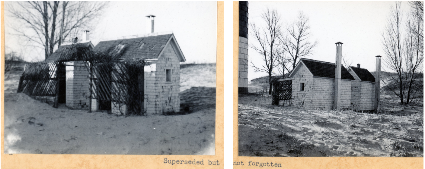
Figure 1B-73: Photos of the two privies located east of the dwelling.
