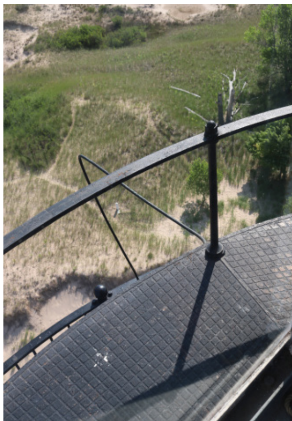
Figure 1D-302 Metal railing around the perimeter of the Lantern Deck.
