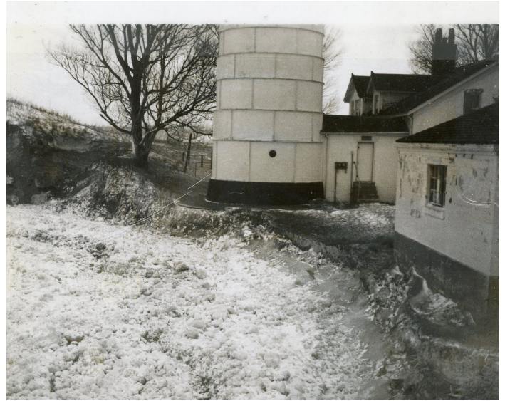
Figure 1B-84: 1978 photo showing shoreline erosion up to concrete sidewalk around the tower base and near the north side of the fog signal control building. The handwritten caption on the back of the photos says, "Photo taken from high ground west of compressor bldg."
