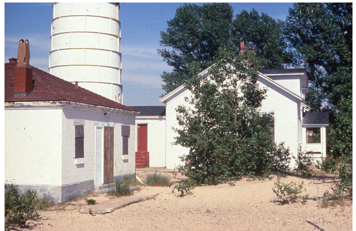
Figure 1C-05: Circa late 1970s photo of the Keepers' Dwelling.
