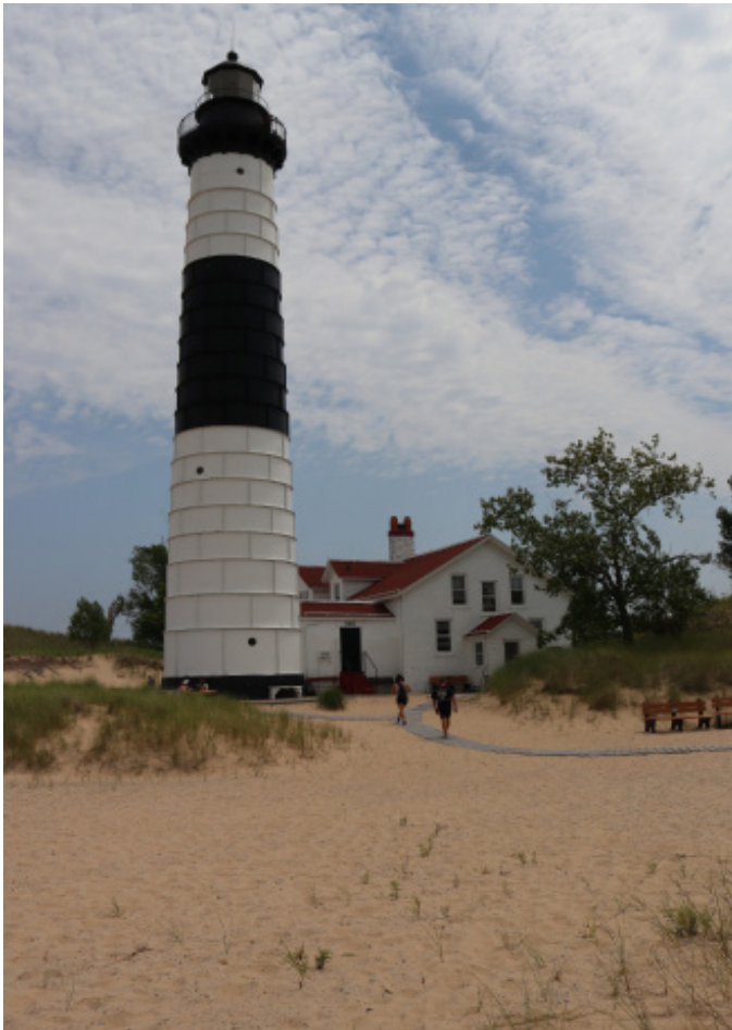
Figure 1D-245 West elevation of the Light Tower.
